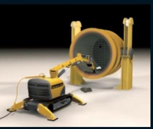
We start by breaking loose the refractory in the lower part of the ladle. We remove the bricks inwards, creating a V-shape.
