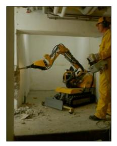
Despite the small size the Brokk 40 is a machine with power and capacity. This means fast and rational demolition in e.g. cramped basements.
