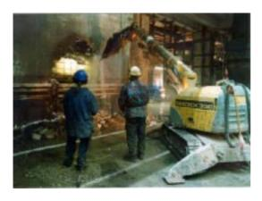
A paper mill is being remodelled and modernised, requiring the tear down of heavily reinforced walls and foundations - a typical Brokk 330 job.
