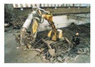
The concrete crusher offers a quiet and vibration-free alternative to the hydraulic breaker for demolition applications.
